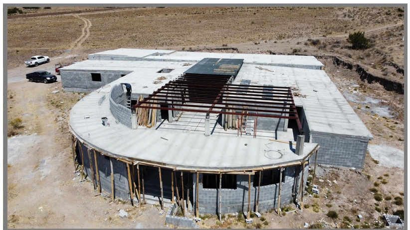
Construction progress being made on the new hospital near Saltillo, Mexico
