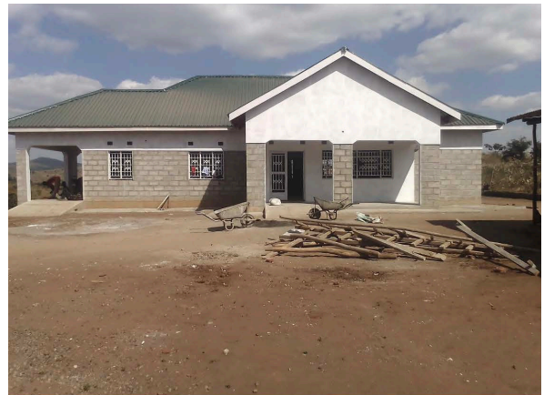
Chipande Health Clinic under construction and nearly completed
